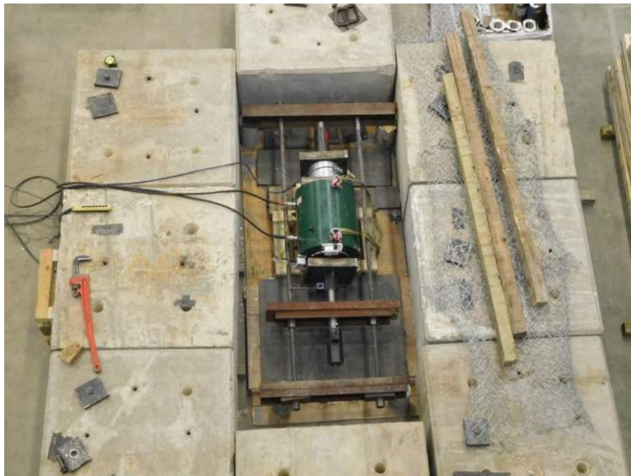
Figure 4.3-2 – The end nut test set-up located in a “concrete block box” for safety.
