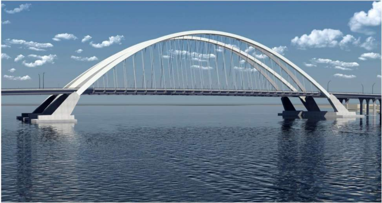
Figure 1-1 - Overall elevation view of the new I-74 twin basket-handle, through arch bridges over the Mississippi River.
