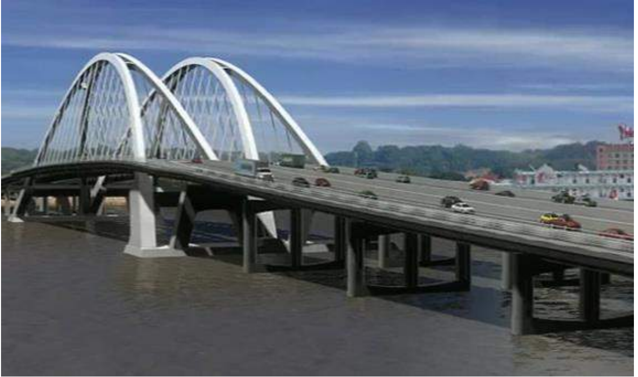
Figure 1-2 - Approach view of the bridges
