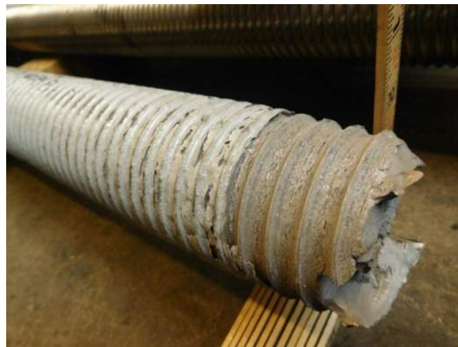
(b) Side view showing loss of the galvanized coating.
