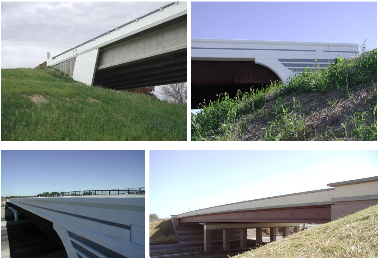
Figure 9.5.3.1. Bridges with long, slender appearance
