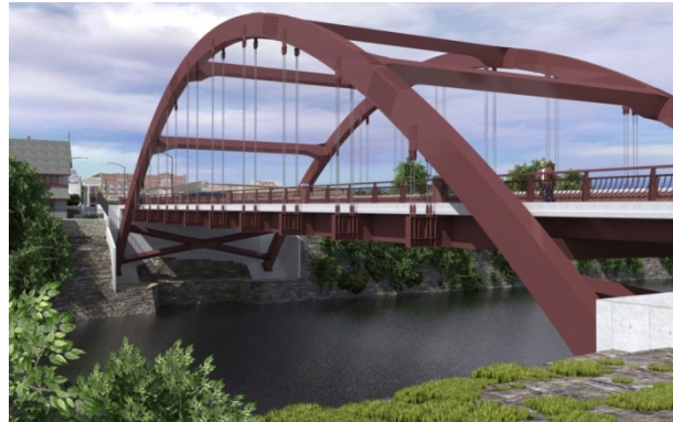
Figure 2.3.1-2 Replacement Steel Arch Bridge
