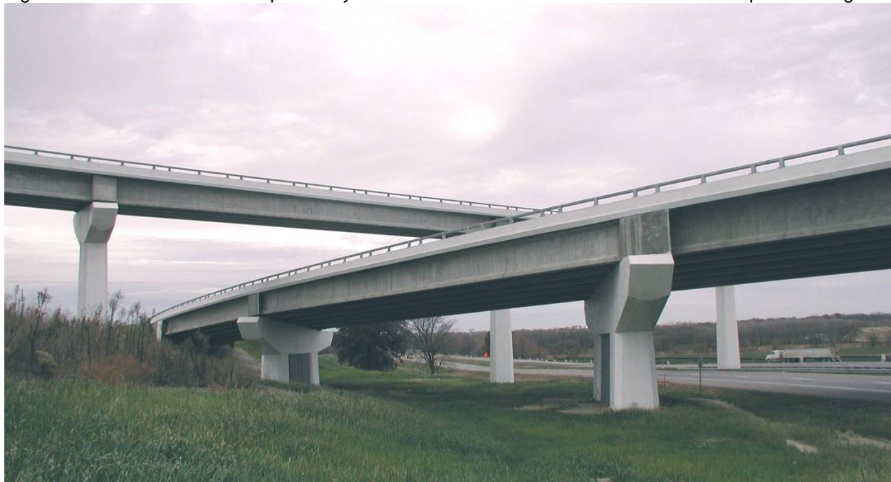
Figure 9.5.3.4. Bridges with minimal column count
