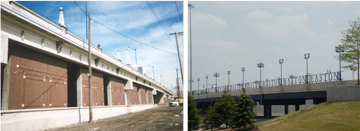
Figure 9.5.3.7-1. Bridges with ineffective bolt-on aesthetic details
