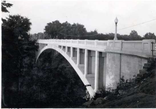
Figure 2.3.1-1 Original Concrete Arch Bridge
